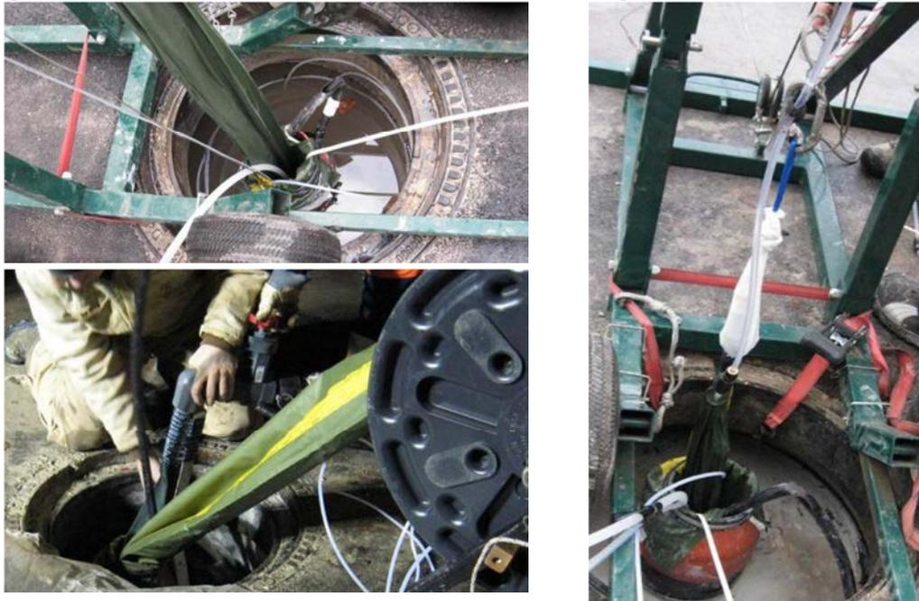
Figure 29: installation of the FACT liner in chalk
