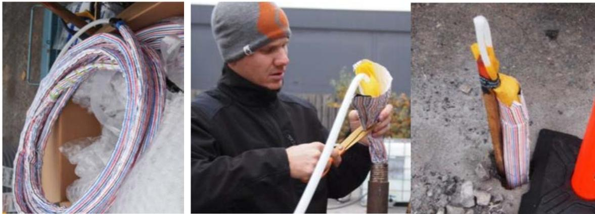
Figure 28: FACT installation; left: FACT material; middle: cutting end of installed FACT, right: installed FACT
